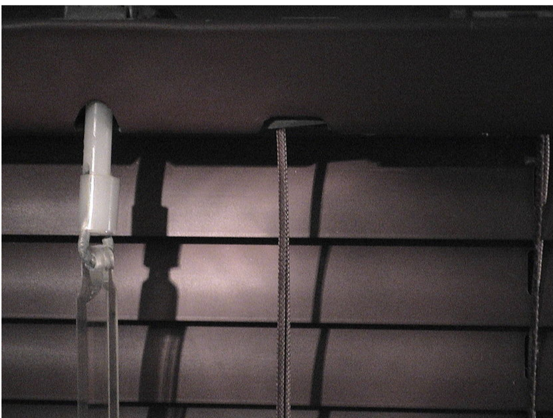
Detail of turning rod (blind stick) attachment on miniblinds
